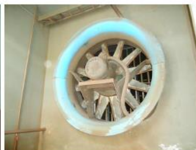
CENTRAL DE CLIMAT. - VENT. AXIAL
