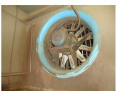
CENTRAL DE CLIMAT. - VENT. AXIAL
